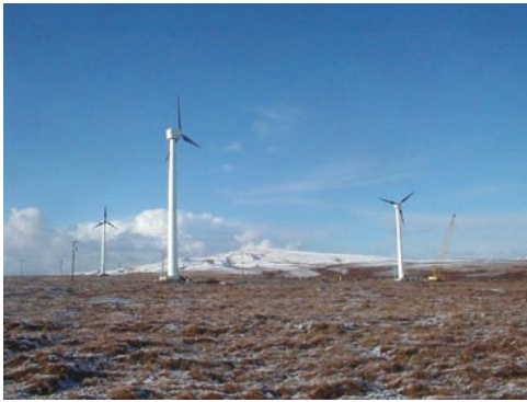
Fig. 1: Operational wind towers.
