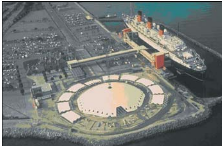
Fig. 6: The “Spruce Goose” dome during erection (Long Beach, California)
