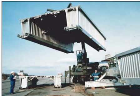
Fig. 13: The German military bridge: erection phases
