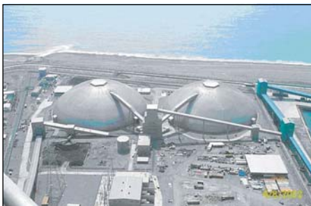
Fig. 7: Aluminium domes for coal storage plant
