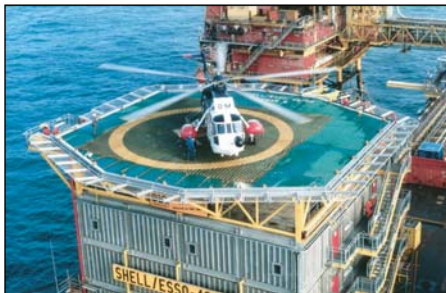
Fig. 11: A structural off-shore application: helideck
