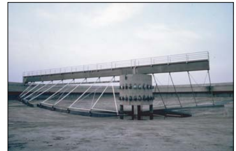
Fig. 10: The sewage plant pool of Po-Sangone (Torino, Italy)
