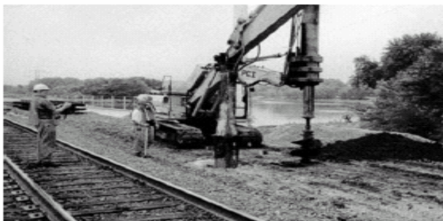
Fig-6: Work for providing stone column
