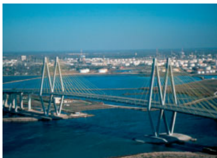
Fig. 26. Houston Ship Channel Crossing, TX, USA
