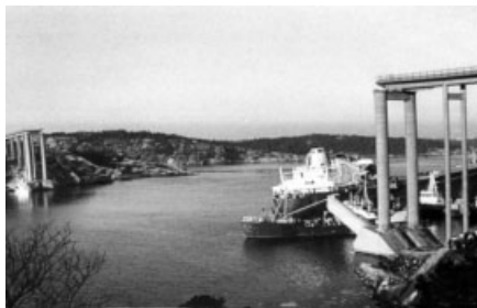
Fig. 15. Old Tjörn Bridge after ship collision
