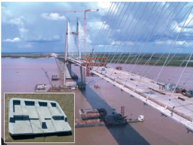
Fig. 40. Rosario-Victoria Bridge, construction of protection
