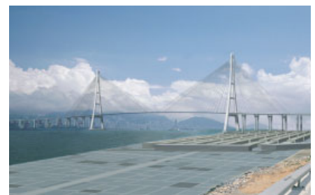
Fig. 20. Stonecutter Bridge, Hong Kong, LAP's 2nd prize design
