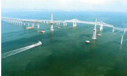
Fig. 36. Sunshine Skyway Bridge, dolphin protection
