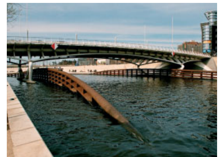
Fig. 28. Crown Prince Bridge, Berlin, Germany
