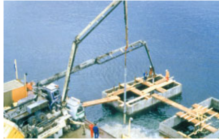
Fig. 51. Helgeland Bridge, construction of solid foundations
