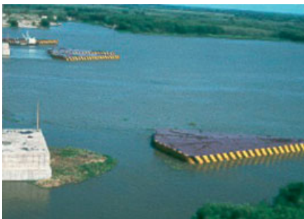
Fig. 33. Zarate Brazo-Largo Bridge, floating protection
