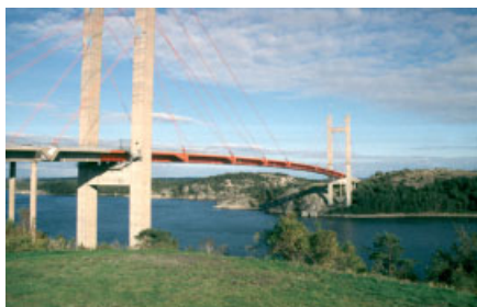
Fig. 16. New Tjörn Bridge, Sweden
