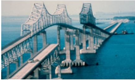
Fig. 35. Sunshine Skyway Bridge, Tampa, FL, USA, collapsed bridge
