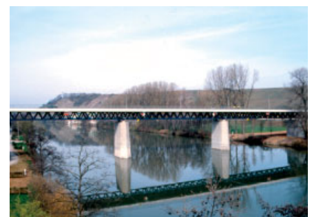
Fig. 30. Bridge over Neckar, Kirchheim, completed bridge
