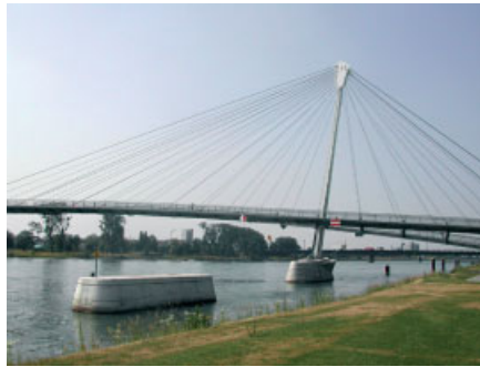
Fig. 43. Rhine Bridge Kehl, Germany, Side Span Protection
