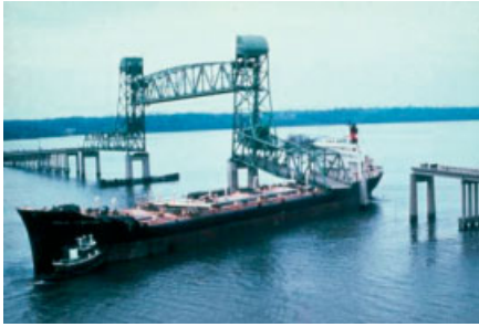
Fig. 42. Ship collision with side span of Benjamin Harrison Bridge, USA
