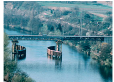
Fig. 29. Bridge over Neckar, Kirchheim, Germany, during construction
