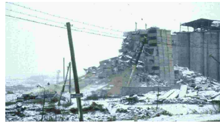
Fig. 13. Damaged grain storage complex and spilled out grains due to 1988 Spitak, Armenia earthquake (Photograph by C. J. Langer; JAMA 2007)
