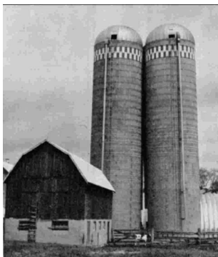
Fig. 5. Leaning twin silos due to nonuniform settlement in zone of overlapping pressure bulbs (Bozozuk 1976, ASCE)
