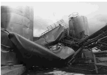
Fig. 12. Collapse of stainless steel milk silos during 1987 Edgecumbe, New Zealand earthquake (CAE 2007, with permission)
